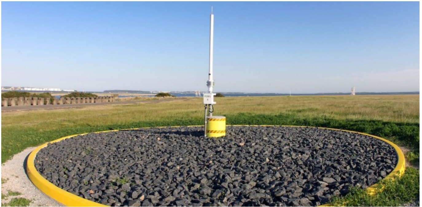
GBAS GPS antenna at Sydney Airport.
