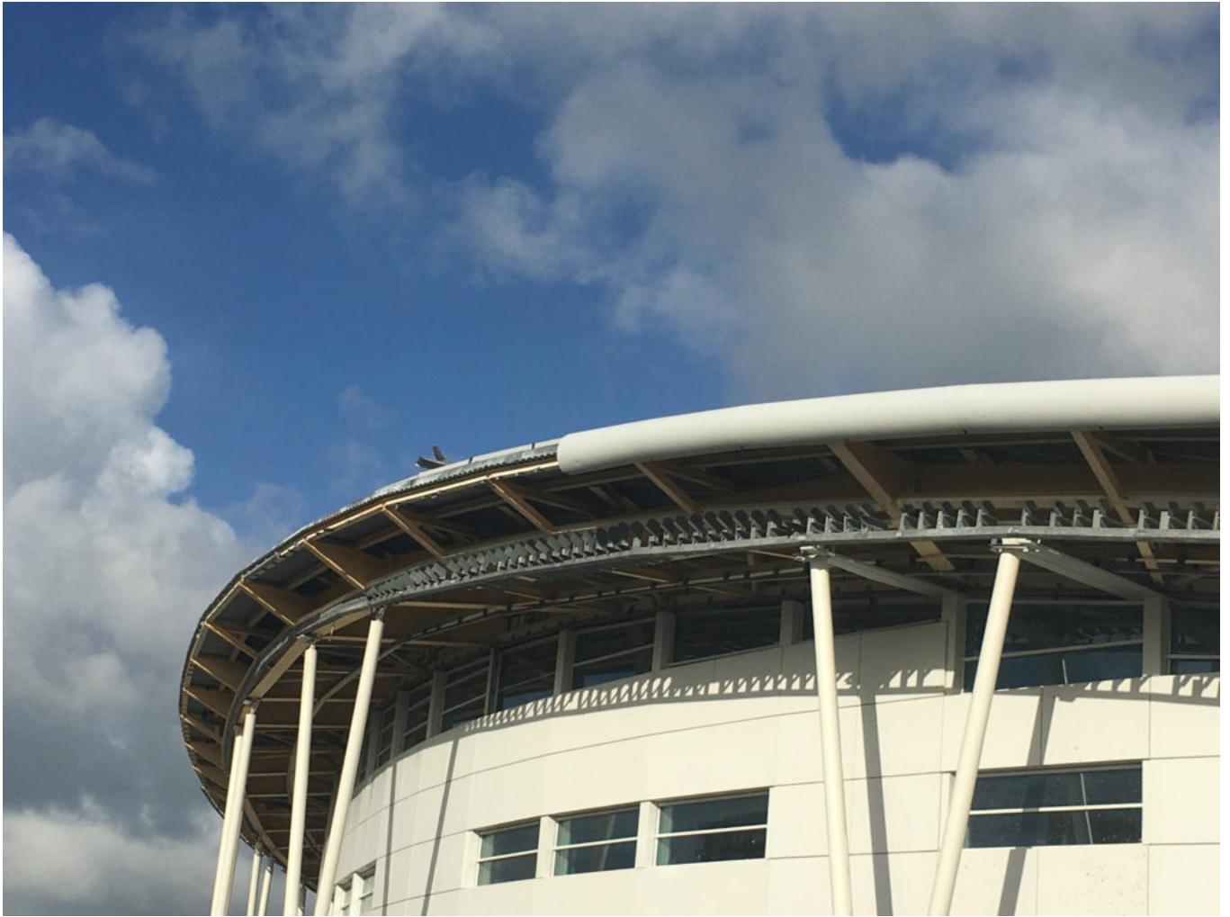
Roof Repairs are Ongoing
