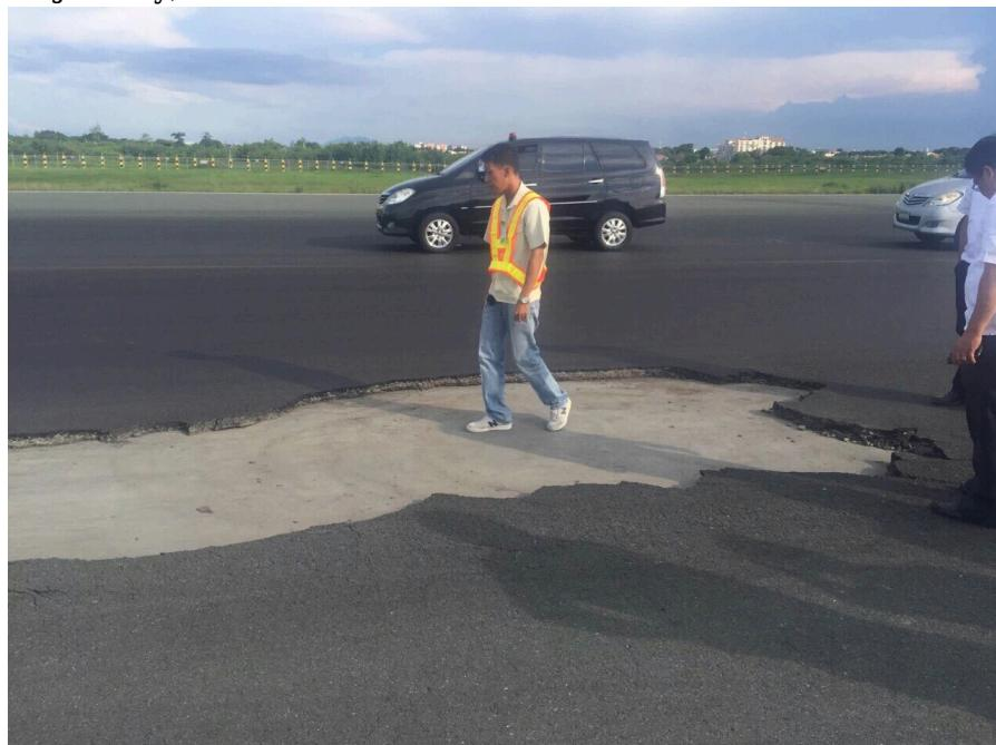
The main runway at RPLL/Manila, RWY 06/24, was closed on Monday 18JUL after heavy rain caused large chunks of asphalt to disintegrate. One of the last aircraft to land, shown below, suffered damage to an inboard flap section.
