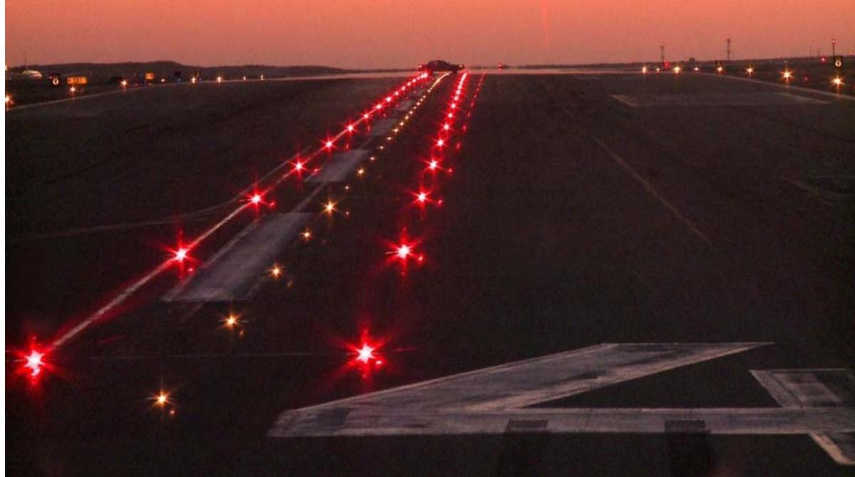
As you may know, the FAA is working on Runway Status Lights (RWSL). It's a new system that's live at 20 airports in the US. Basically, you get a nice set of red lights (embedded in the ramp) that tell you whether it's safe or not to proceed. These lights are installed (or placed or located) at the entrance of the runway and at the start of takeoff. If any of these lights are red, you don't go. Simple as that.
