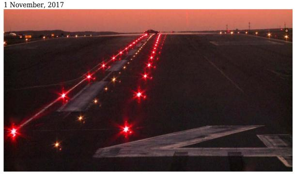
As you may know, the FAA is working on Runway Status Lights (RWSL). It's a new system that's live at 20 airports in the US. Basically, you get a nice set of red lights (embedded in the ramp) that tell you whether it's safe or not to proceed. These lights are installed (or placed or located) at the entrance of the runway and at the start of takeoff. If any of these lights are red, you don't go. Simple as that.
