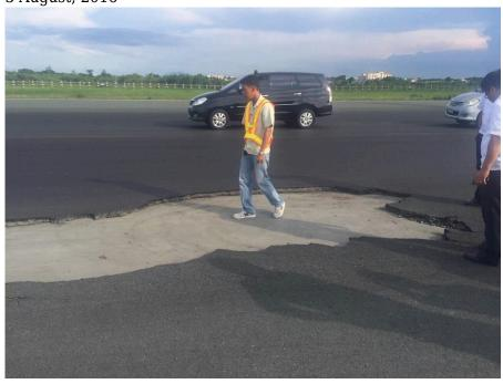
The main runway at RPLL/Manila, RWY 06/24, was closed on Monday 18JUL after heavy rain caused large chunks of asphalt to disintegrate. One of the last aircraft to land, shown below, suffered damage to an inboard flap section.
